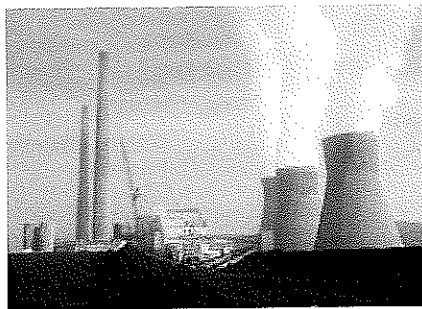
Figure 5. Coal Burning Power plant
