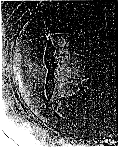
Figure 13.6 Collapsed scotch marine boiler's corrugated furnace caused by scale and dry firing. (Courtesy Royal Insurance Co.)
