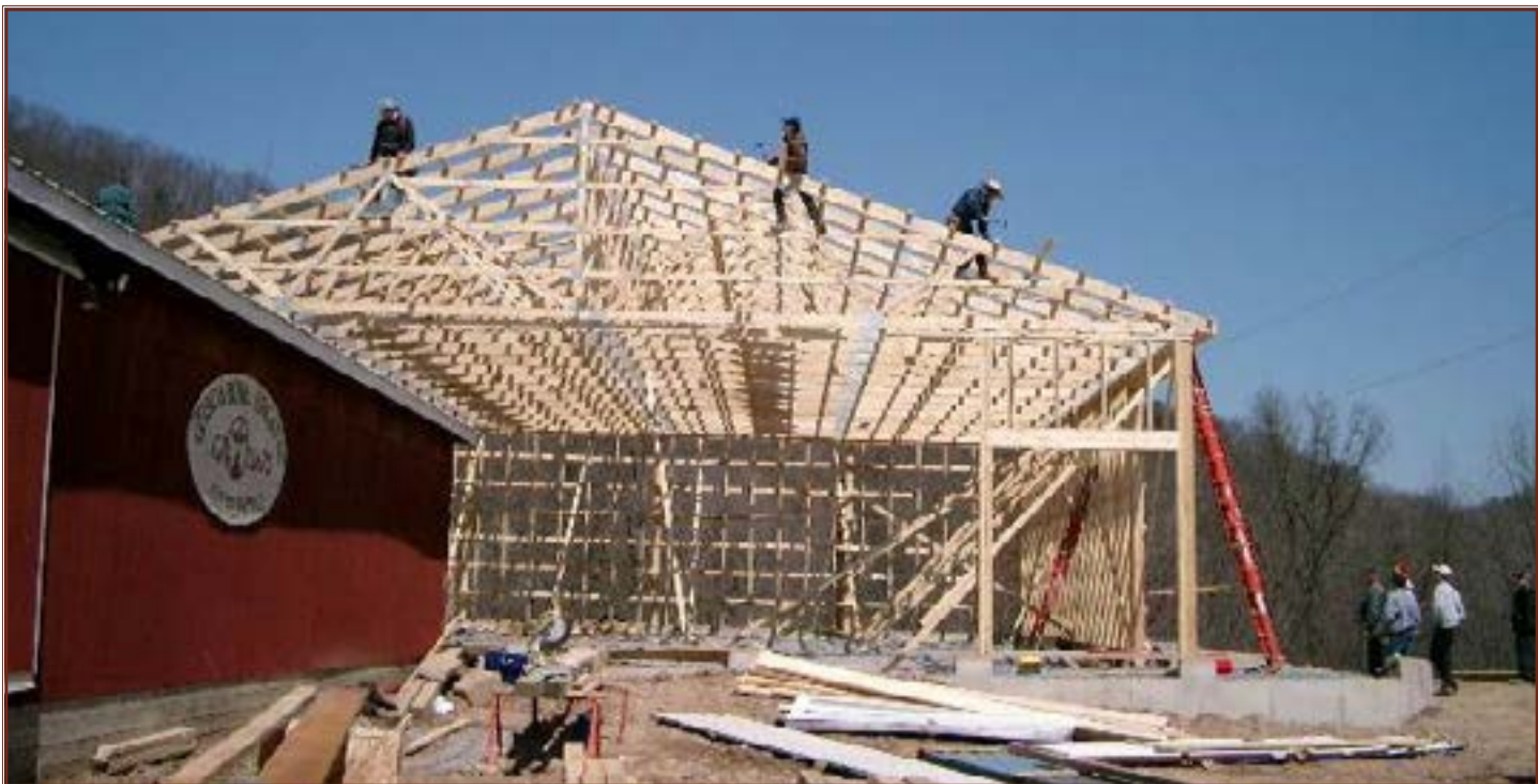
Construction of 2004 addition.
