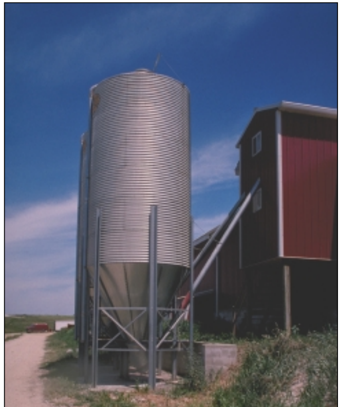
Large-capacity feed tanks provide a continuous supply of feed to each layer house. (CD 8202 3241 1143-96)
